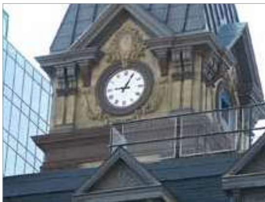
The Halifax City Hall clock has remained stuck at 9:05 since the day of the explosion.
