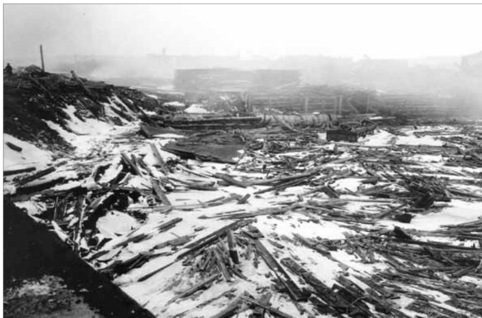
Piers 7, 8, and 9 were completely obliterated by the blast.
